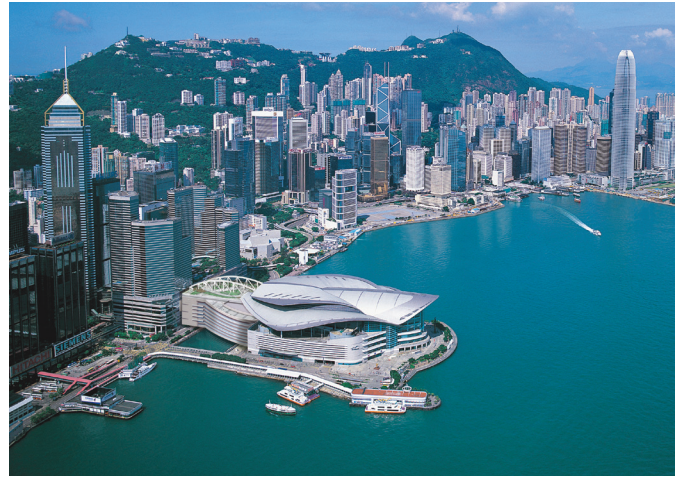
Harbour-side Hong Kong Convention and Exhibition Centre extension.
