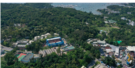
New quarantine facilities were constructed in Sai Kung Outdoor Recreation Centre in March.
