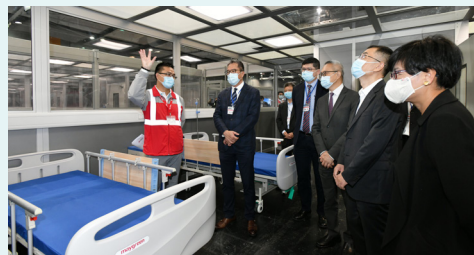
Inspection of the negative pressure ward of the community treatment facility at AsiaWorld-Expo
